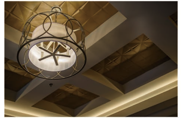
Ceiling in Rest room/ Code :HS-505b
